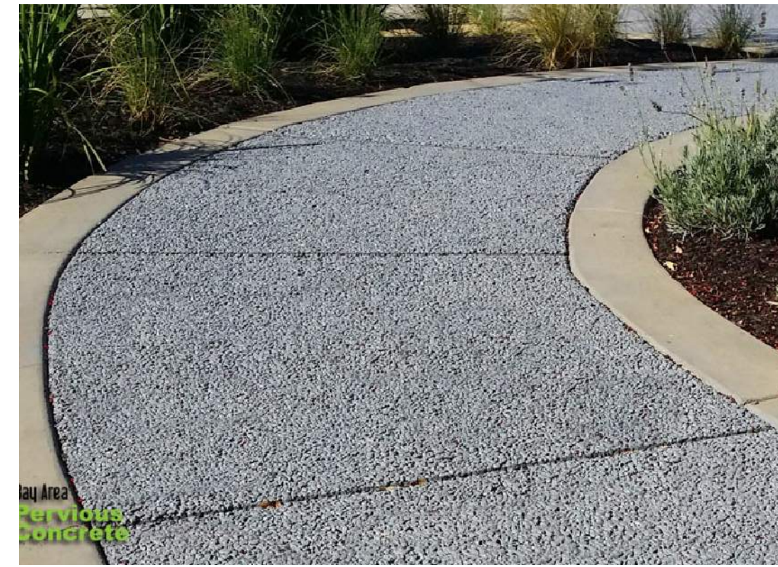
7 | PERMEABLE CONCRETE NTS
