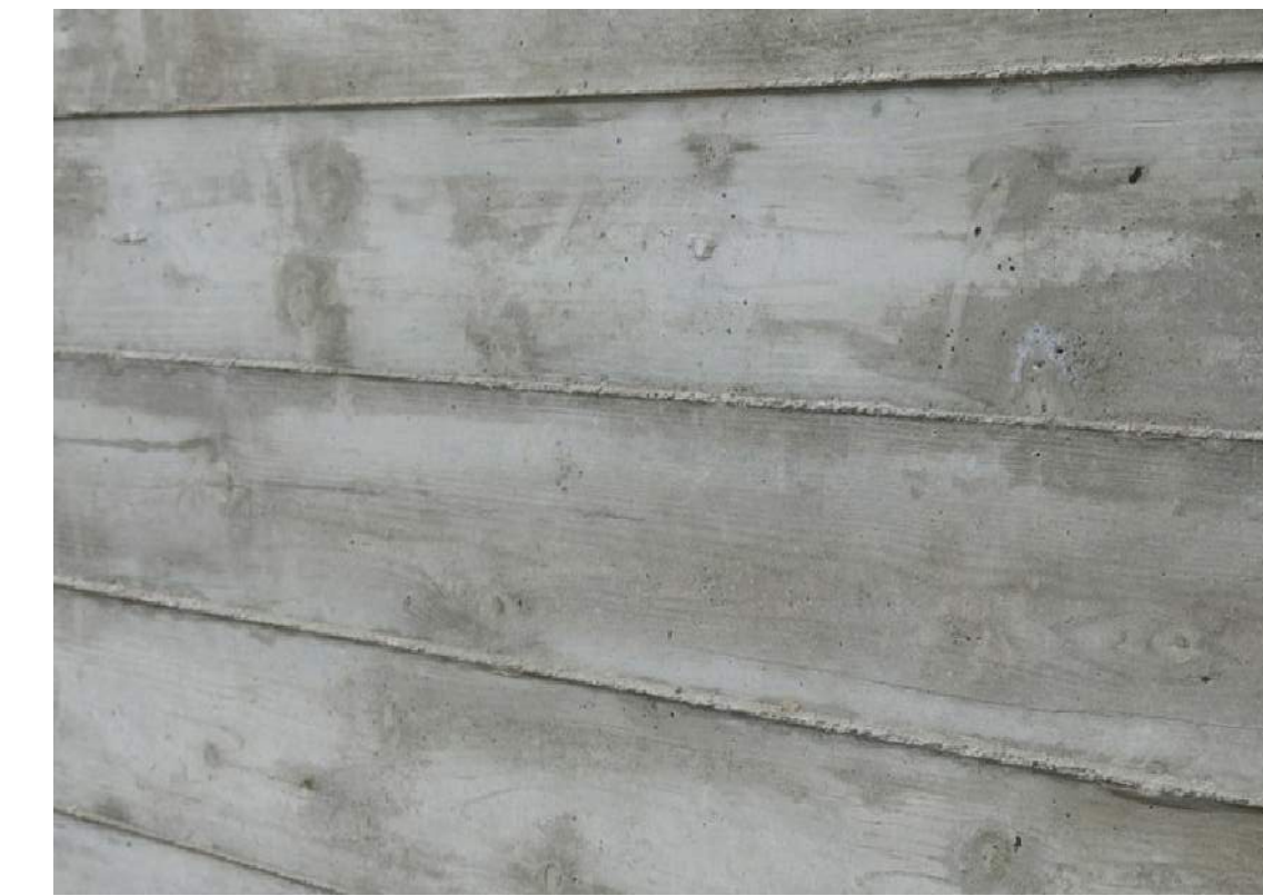
4 | BOARD FORMED CONCRETE NTS
