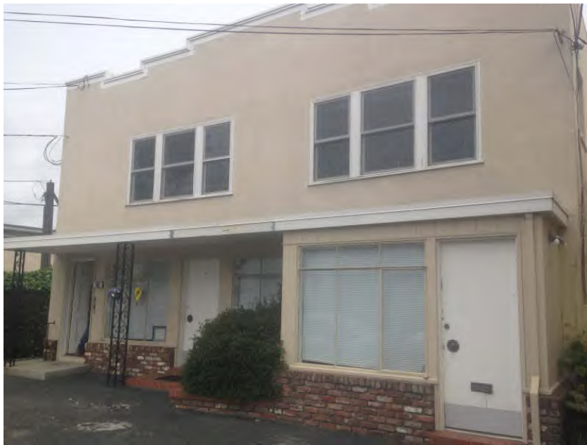
Photo 1. 108 Myrtle Road - View looking northeast toward property showing vacant office space and second floor residential units. Photograph taken April 26, 2017.
