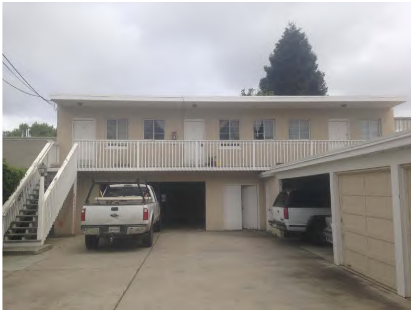
Photo 2. 108 Myrtle Road - View looking east showing carports, storage units, and second floor residential units in northeast portion of property. Photograph taken April 26, 2017.
