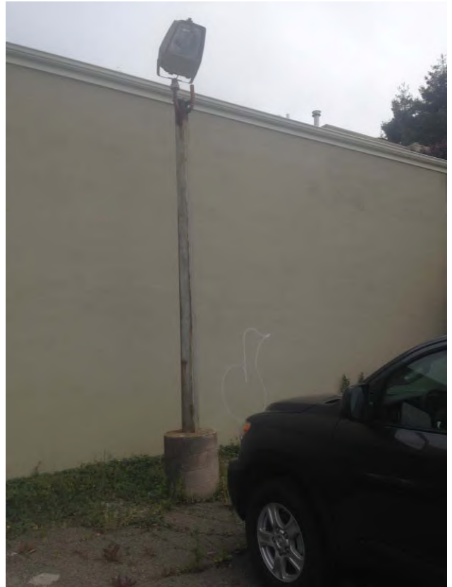
Photo 2. 112-114 Myrtle Road - View of utility pole located along eastern property boundary. Photograph taken April 26, 2017.
