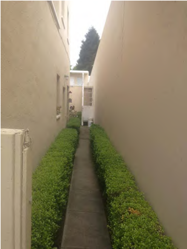
Photo 1. 108 Myrtle Road - View looking northeast showing alley along southeast property boundary. Photograph taken April 26, 2017.
