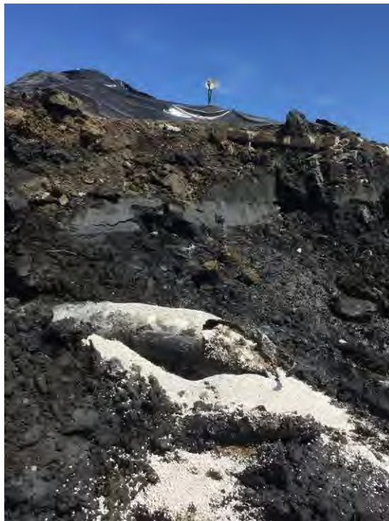
Photograph 4 (13 June 2019): Section of pipe with semi-solid petroleum product with absorbent material prior to removal.
