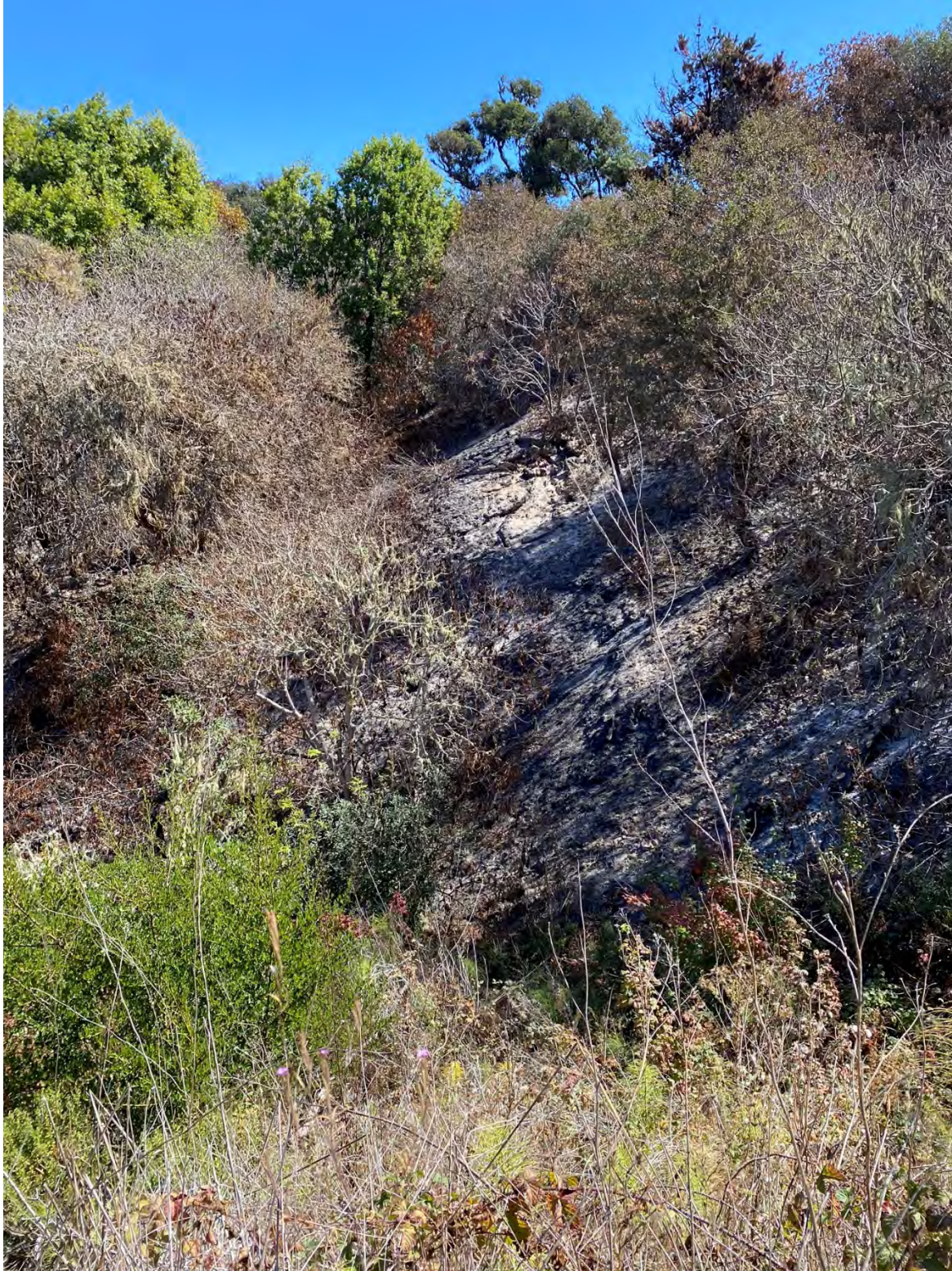
Photograph 9: Ano Nuevo SP, SR-1, facing east from NB shoulder of SR-1; shows CZU Lightning Complex fire damage on hillside immediately adjacent to project footprint [09/24/2020]
